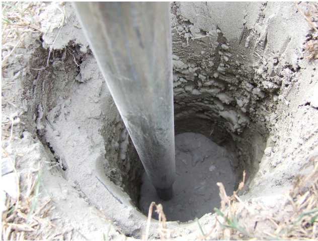
Figure 6. High tunnel poles set in concrete. (Photo by Lynn Brandenberger)
