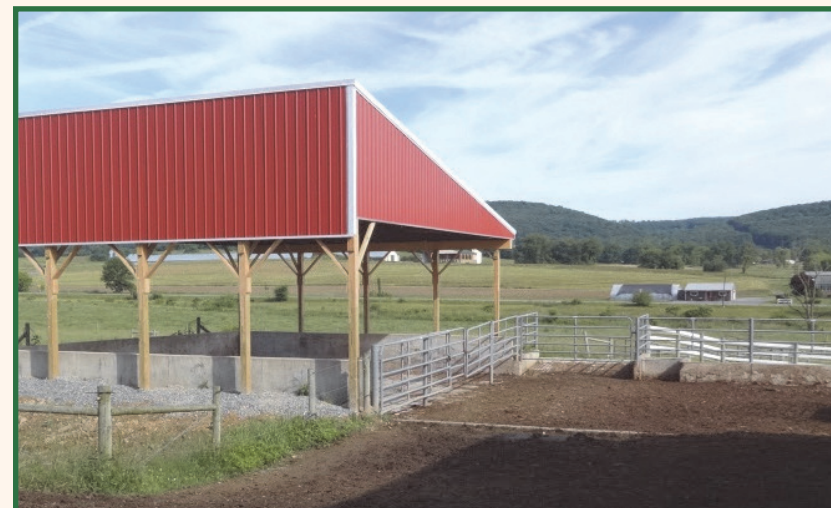
Roofed Concrete Manure Stacking area
