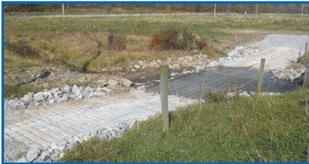
Cattle Crossing to protect stream beds and stream banks
